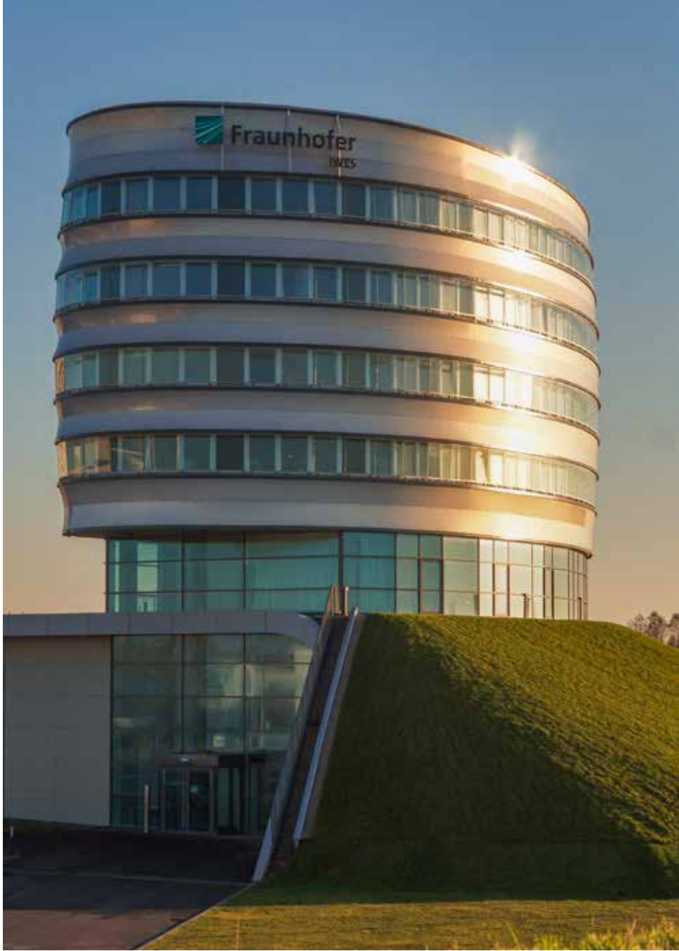
1 Engineering building in Bremerhaven, built on a terp.
